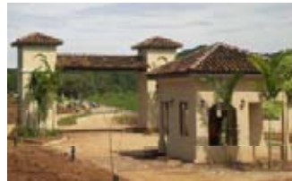
The main entrance to Rancho Villa Real
